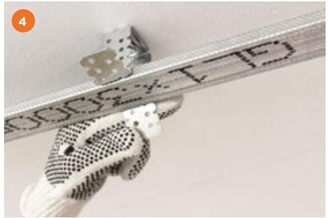
The protruding legs of each bracket are bent to sit back from the channel face. Additional angle or supplementary framing is installed if required to support fixtures.
