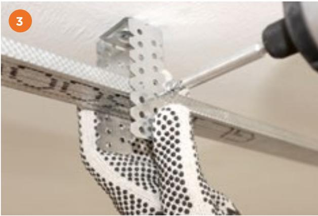
Gypframe GL1 Lining Channels are located into the perimeter track and each leg of the Gypframe GLB85 or GLB135 Brackets are screw-fixed to the Gypframe GL1 Lining Channels with Gyproc Waferhead Screws.
