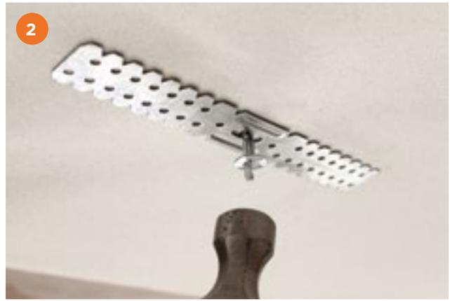
Gypframe GLB85 or GLB135 Brackets are fixed to the soffit at the required centres using Gyproc Wedge Anchor.
