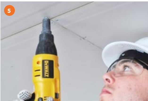
Gyproc Boards are fixed to the Gypframe GL1 Lining Channels to form single or multi-layer linings as specified.
