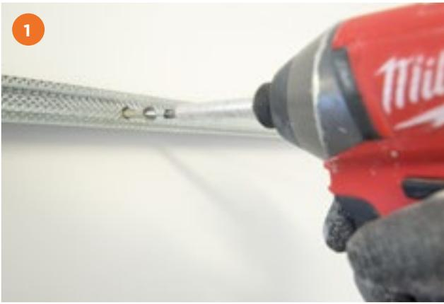
Gypframe GA1 Perimeter Angle is fixed to the wall at maximum 600mm centres using Gyproc Hammer Fix Anchor.
