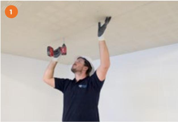
Install Gyproframe ceiling framework as described in the Gyproc mf ceiling section ensuring that Gyproframe MF5's are installed at 600mm centres. Set out the ceiling ensuring Gyptone boards are installed perpendicular to the MF5's and Gyptone patterns are aligned.
