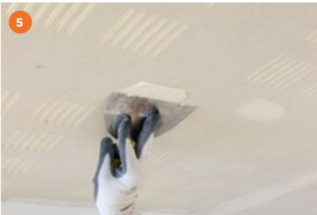
Screw heads are then filled with Gyproc Joint Compound and sanded back to a smooth finish.
