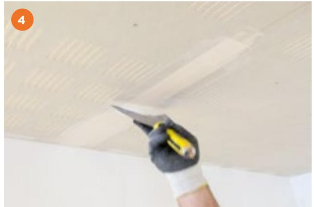
When set, sand if necessary and apply a further coat of Gyproc Jointing Compound and trowel flat taking care not to fill the perforations in the board. Lightly sand to a flat finish and dust off.
