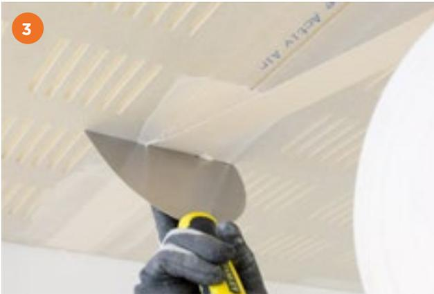
Gyptone BIG boards have all four edges tapered to allow for true flat joints to be created at each board interface to give a perfectly flat finished ceiling. Bed Gyproc Paper Tape firmly into Gyproc Jointing Compound and bulk fill the taper edge joints.
