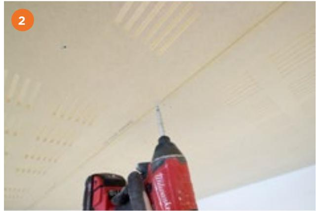
Fix Gyptone BIG boards using 25mm Gyproc Drywall Screws. Screws are inserted at 200mm centres, 15mm from board edges and 50mm from corners.
