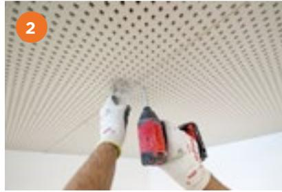
Fix Rigitone boards using 25mm Gyproc Drywall Screws at a maximum of 170mm centres. Screw fix the board perimeter prior to fixing the field of the board.
