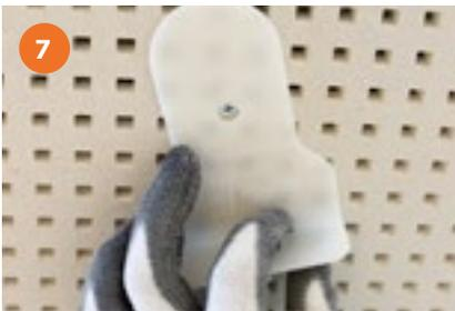
Screw heads are then filled with Gyproc Joint Compound using the Rigitone screw head template to help ensure no jointing compound enters into the perforations of the board.
