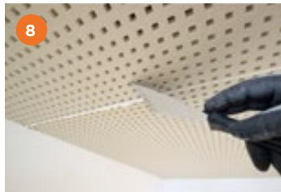
Once the Rigitone Mix between the boards has begun to harden, remove any excess carefully using the Rigitone scraper. Pass the scraper back over the joints in the other direction to smooth the surface.
