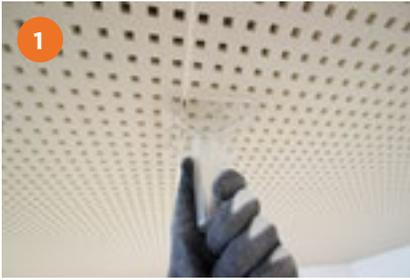
Install the Gypframe ceiling framework as described in the Gyproc MF ceiling section ensuring that Gypframe MF5's are installed at approximately 330mm centres - see Table 1 for guidance. Set out the ceiling ensuring Rigitone boards are installed perpendicular to the MF5's and the Rigitone patterns are aligned using the Rigitone Installation Kit to correctly space the boards.
