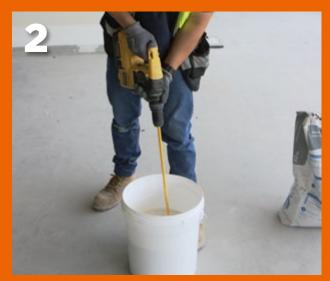
Mix until a smooth consistency is achieved. Best mixed using a power mixing tool at low speed, max 200rpm.
