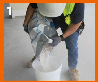
Add 10kg of Gyproc Plasterboard Adhesive gradually to 3.2 litres of clean water in a clean bucket. Leave for approximately 3 minutes before mixing well.
