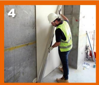
Position the plasterboard in place, tapping the board back firmly using a straight-edge until it aligns with the ceiling and floor chalk lines.
