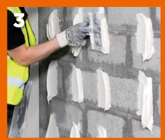
Trowel apply adhesive to form dabs 50mm to 75mm wide and about 250mm long. Position dabs of Gyproc Plasterboard Adhesive in three vertical rows to receive the first board. Apply a continuous band of Gyproc Plasterboard Adhesive at skirting level.
