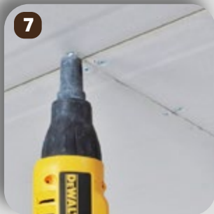
Fix Plasterboard
