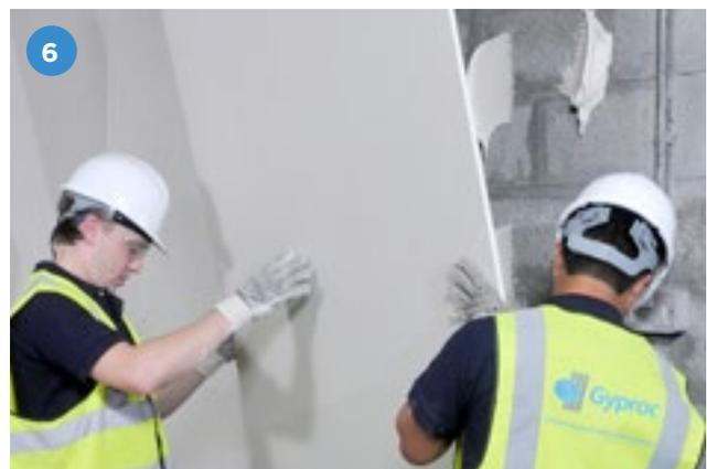
6 Position the boards with the bottom edge resting on plasterboard packing strips. Boards are 'tapped' into position, lifted tight to the ceiling using a footlifter and supported until the adhesive sets. Further boards are installed, lightly butted together, to complete the lining.
