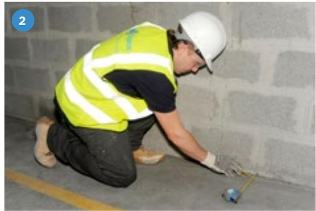
2 Mark the wall with lines at 1200mm centres to indicate board positioning.
