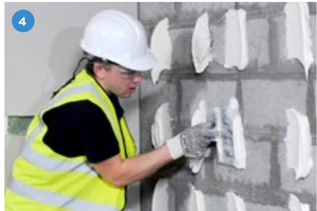
4 Commence drylining from a window / door reveal or internal angle, apply adhesive dabs in three or four rows (as appropriate) to receive the first board, together with intermediate dabs at ceiling level and a continuous band of adhesive at skirting level.
