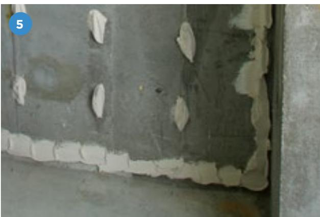
5 A continuous fillet / ribbon of Gyproc Plasterboard Adhesive is applied to the wall perimeter and around all services and openings as board fixing proceeds. This is important if the lining is designed to act as an air barrier to achieve building airtightness.
