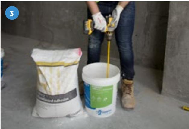
3 Take a clean bucket and add approximately 10kg of Gyproc Plasterboard Adhesive gradually to 5 litres of clean water. Leave for 3 minutes before mixing. Mix until a smooth consistency is achieved. We recommend using a power mixing tool at speed not exceeding 200rpm.
