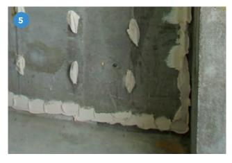
A continuous fillet / ribbon of Gyproc Plasterboard Adhesive is applied to the wall perimeter and around all services and openings as board fixing proceeds. This is important if the lining is designed to act as an air barrier to achieve building airtightness.
