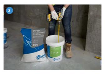
Take a clean bucket and add approximately 10kg of Gyproc Plasterboard Adhesive gradually to 5 litres of clean water. Leave for 3 minutes before mixing. Mix until a smooth consistency is achieved. We recommend using a power mixing tool at speed not exceeding 200rpm.
