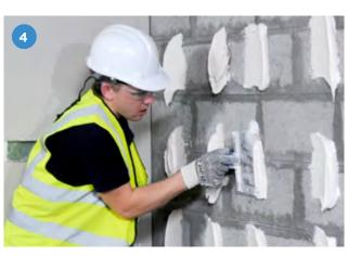
Commence drylining from a window / door reveal or internal angle, apply adhesive dabs in three or four rows (as appropriate) to receive the first board, together with intermediate dabs at ceiling level and a continuous band of adhesive at skirting level.
