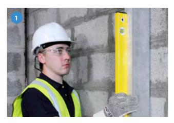
Mark setting out lines on the floor and ceiling allowing for high spots, a minimum 10mm & maximum 25mm drylining cavity and the thickness of board.
