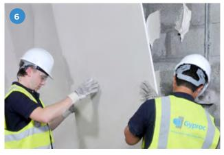
Position the boards with the bottom edge resting on plasterboard packing strips. Boards are 'tapped' into position, lifted tight to the ceiling using a footlifter and supported until the adhesive sets. Further boards are installed, lightly butted together, to complete the lining.
