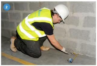
Mark the wall with lines at 1200mm centres to indicate board positioning.
