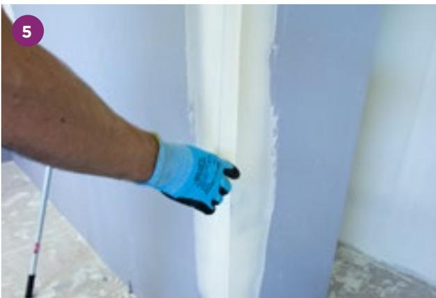
For external corners, repeat step 1 to 4 using Habito 83 Flex, Levelline Flex or Gyproc Drywall Corner Bead for corner reinforcement. Use Gyproc Edge Bead to protect cut ends of boards.
