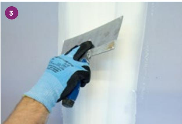
Trowel apply a second coat of jointing compound feathering out beyond the previous application and spot the screws head. Allow to dry.
