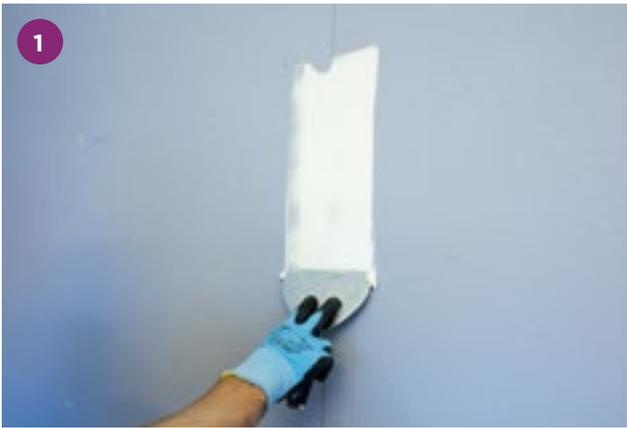
Apply Gyproc Jointing Compound to the board joints and internal corners.
