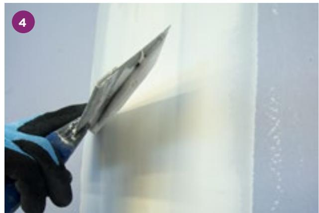
Trowel apply a third coat of jointing compound feathering out beyond the previous application and spot the screws head. Allow to dry.
