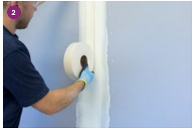
Bed Gyproc or Glasroc X joint tape firmly into the jointing compound.
