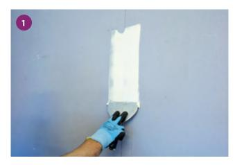
Apply Gyproc Jointing Compound to the board joints and internal corners.
