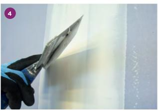
Trowel apply a third coat of jointing compound feathering out beyond the previous application and spot the screws head. Allow to dry.
