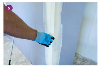
For external corners, repeat step 1 to 4 using Habito 83 Flex, Levelline Flex or Gyproc Drywall Corner Bead for corner reinforcement. Use Gyproc Edge Bead to protect cut ends of boards.
