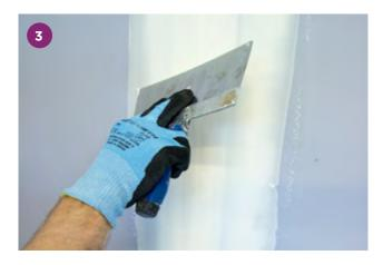
Trowel apply a second coat of jointing compound feathering out beyond the previous application and spot the screws head. Allow to dry.
