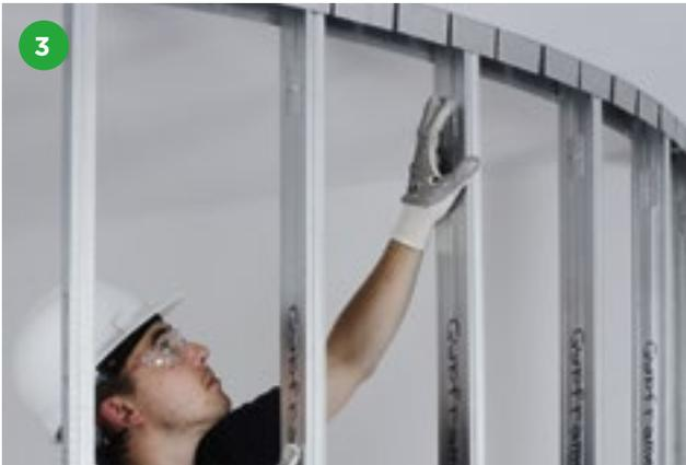
Gypframe studs are fitted vertically within channel sections, and to abutments to form the framework.
