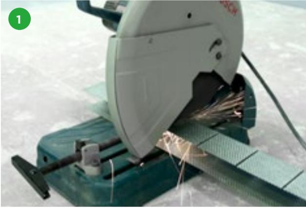
Gypframe Extra Deep Channel is cut and bent on-site to the required radius to achieve a smooth and un-faceted line.
