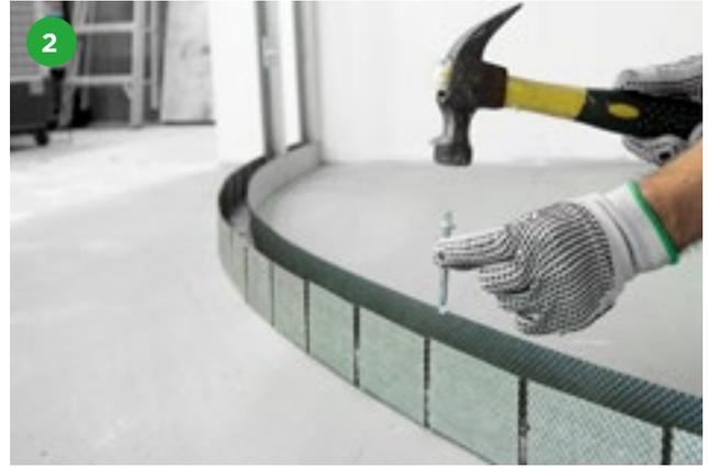
Gypframe Floor & Ceiling channels are fixed to the concrete substrate using Gyproc Wedge Anchors (for fire rated systems) or Gyproc Hammer Fix (for non-fire rated systems).
