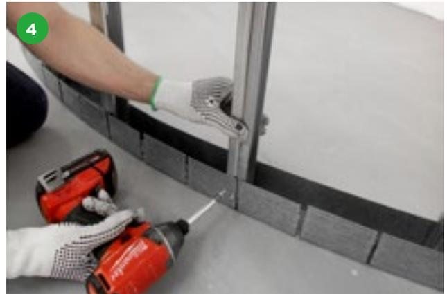
Gypframe studs are fixed into the channel at both head and base and must all face the same way. If a deflection head is required, the studs should not be fixed into the head channel.
