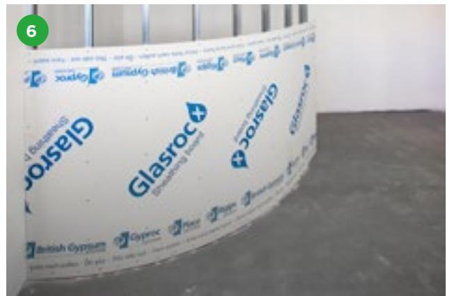
Boards are fixed horizontally. Stagger board joints and avoid vertical joints occurring on the apex of the curve.
