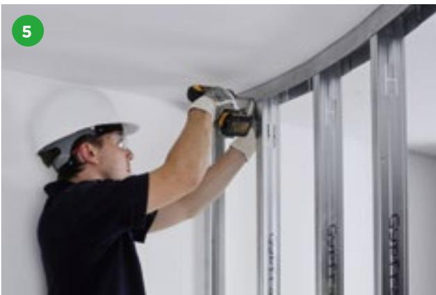
Gyproc plasterboard / Glasroc specialist boards are then fixed to the Gypframe framework with Gyproc Drywall Screws.
