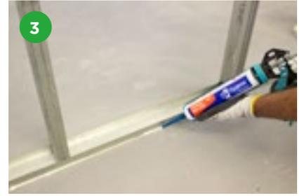
The perimeter of the metal framework is then sealed with Gyproc Sealant for optimum sound insulation performance.
