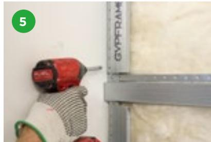
Gypframe RB1 Resilient Bars are installed vertically to abutment and door studs to accept perimeter fixings for the Gyproc plasterboard linings.
