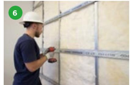
Gypframe RB1 Resilient Bars are fixed across the stud framing and are joined by nesting them together and fixing to Gypframe 'C' Studs using Gyproc Waferhead Screws. Gypframe RB1 Resilient Bars are fixed through the angled flange with the resilient section hanging downward, with the exception of the uppermost and bottommost bar, which are fixed with the resilient section pointing upwards to provide board fixing at the head and additional robustness at the base.
