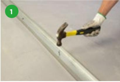
Gypframe Floor & Ceiling channels are fixed to the concrete substrate using Gyproc Wedge Anchors (for fire rated systems) or Gyproc Hammer Fix (for non-fire rated systems). Where Gypframe RB1 Resilient Bars are used to one side only, consider the Gypframe RB1 Resilient Bar dimension of 16mm when setting out.
