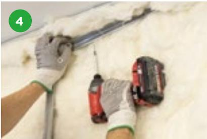
ISOVER Eco APR is added to the partition cavity.
