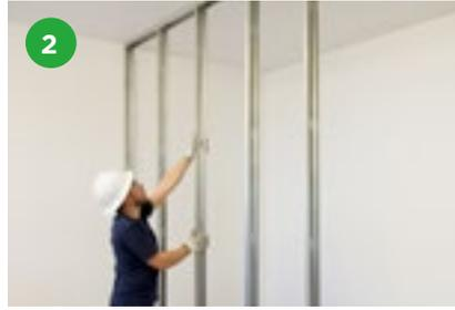
Gypframe 'C' Studs are suitably fixed to abutments and are fitted vertically to a friction fit within the channel sections to form the framework. Studs are fitted to all face the same way.
