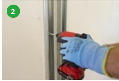
Gypframe 'C' Studs are suitably fixed to abutments.
