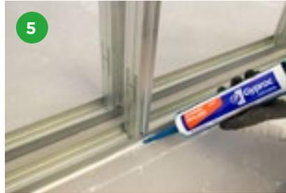
The perimeter of each frame is then sealed with Gyproc Sealant to seal airpaths and to provide optimum acoustic performance.
