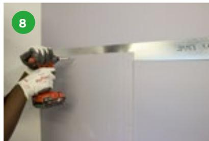
Gypframe GFS1 Fixing Strap to support horizontal board joints in the face layer board.
