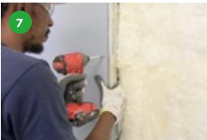
Gyproc plasterboards are fixed with Gyproc Drywall Screws to Gypframe studs. Ensure board joints are staggered between board layers.
