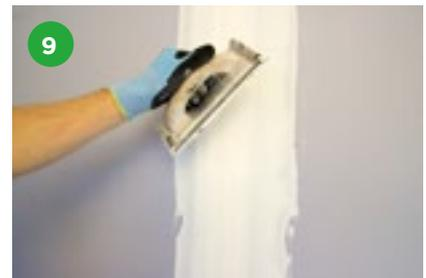
Boards are then taped and jointed using Gyproc Jointing Compound along with Gyproc joint tape and sanded to achieve a smooth finish.
