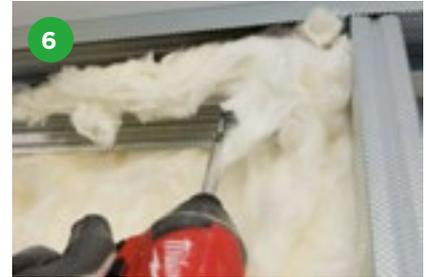
ISOVER Eco APR is added to the partition cavity for increased acoustic performance.
