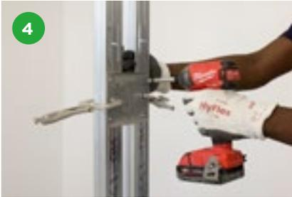
Stud pairs are braced together using appropriate lengths of Gypframe 103 FC 50 Fixing Channel. Use four Gyproc Waferhead Screws per brace, two screws per stud.
