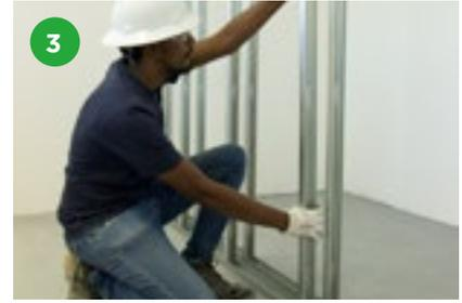
Gypframe 'C' studs are fitted vertically to a friction fit within the both channel sections to form the twin framework. Studs are fitted to all face the same way.
