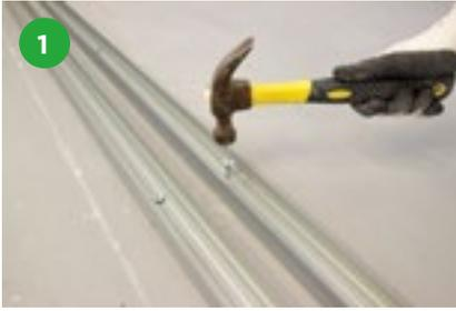
Two rows of Gypframe Floor & Ceiling channels, set out to required dimensions, ensuring a gap between channel, are fixed to the concrete substrate using Gyproc Wedge Anchors (for fire rated systems) or Gyproc Hammer Fix (for non-fire rated systems).
