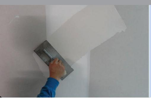
One day course covering all aspects of plaster skimming to plasterboard and other cementitious / gypsum substrates using Gyproc GypFine finishing plasters
